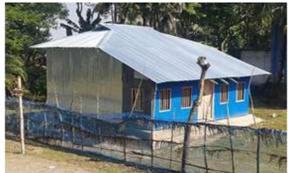
Fig 10: Elongated roof of vernacular house
