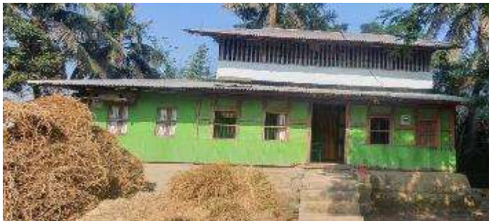
Fig 11: Double storied vernacular house
